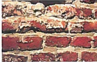
Figure 1: A picture of Madame John's Legacy build in 1788 and the salt damage seen nowadays
