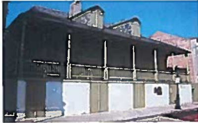
Figure 1: A picture of Madame John's Legacy build in 1788 and the salt damage seen nowadays
